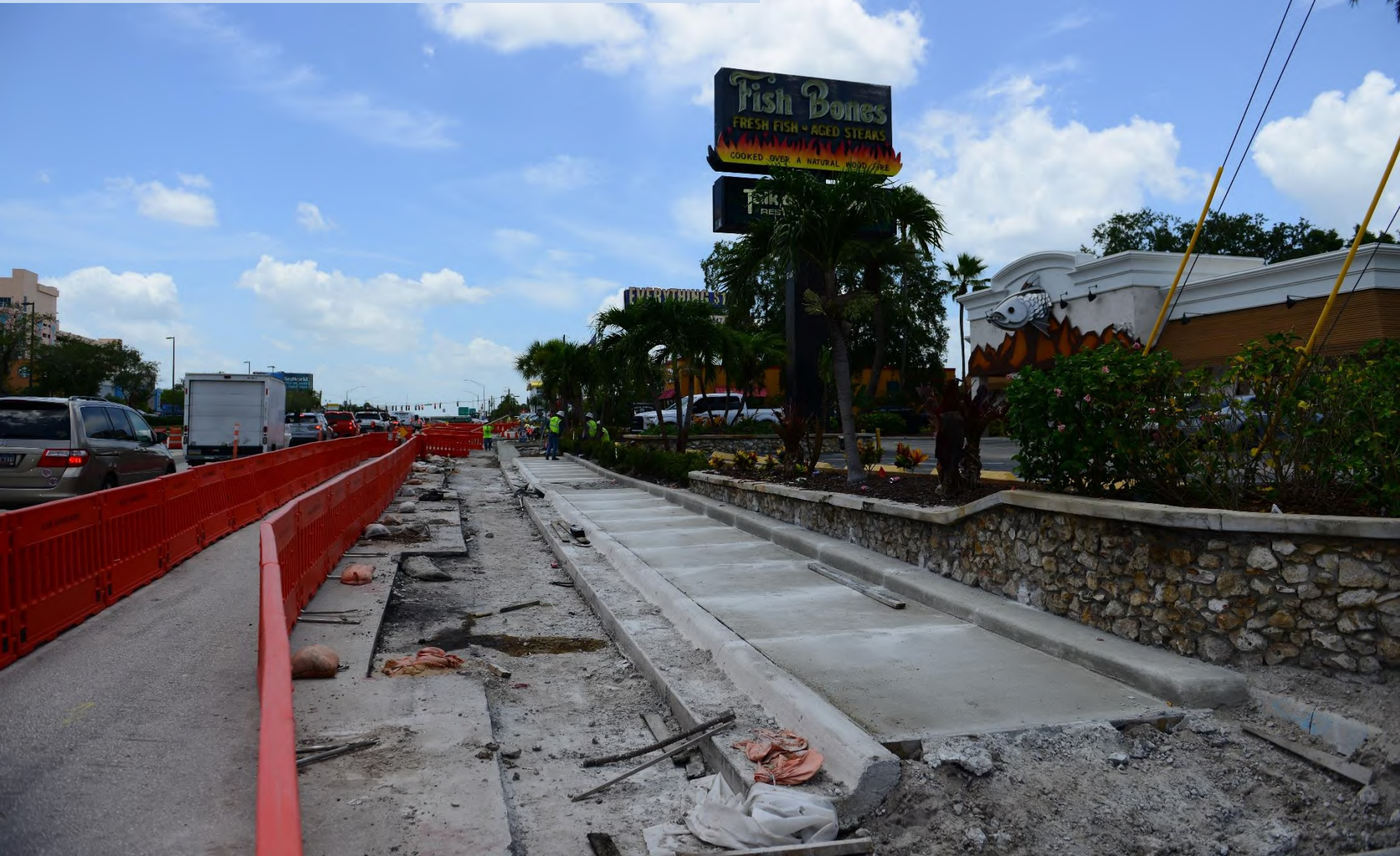
Sidewalk and curb on Sand Lake Rd. near I-Drive
