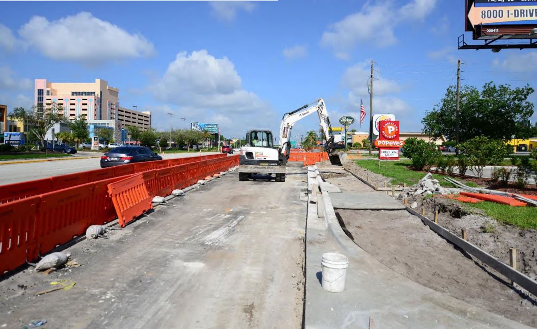
Sidewalk and curb Sand Lake Rd. near I-Drive
