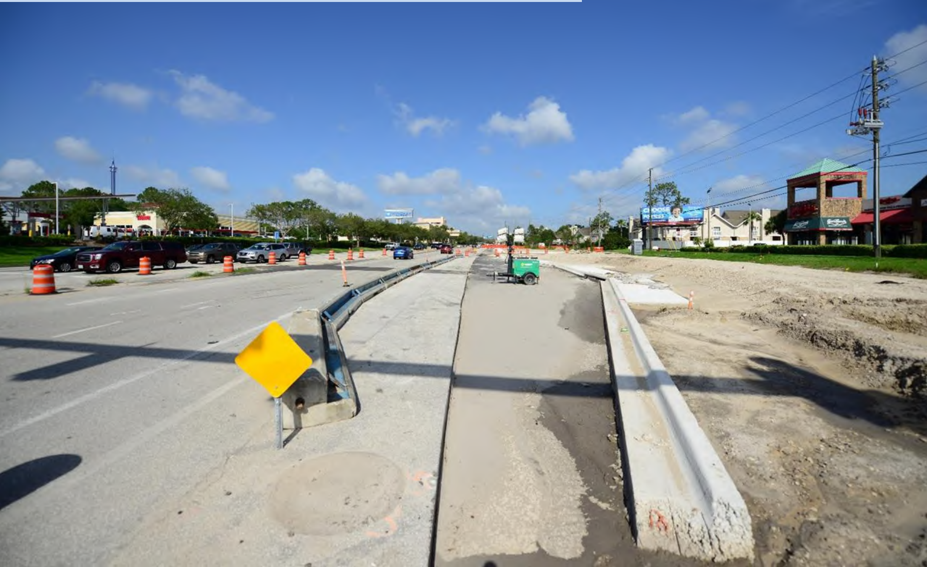
Bus bay construction on Sand Lake Rd. near Universal Blvd.
