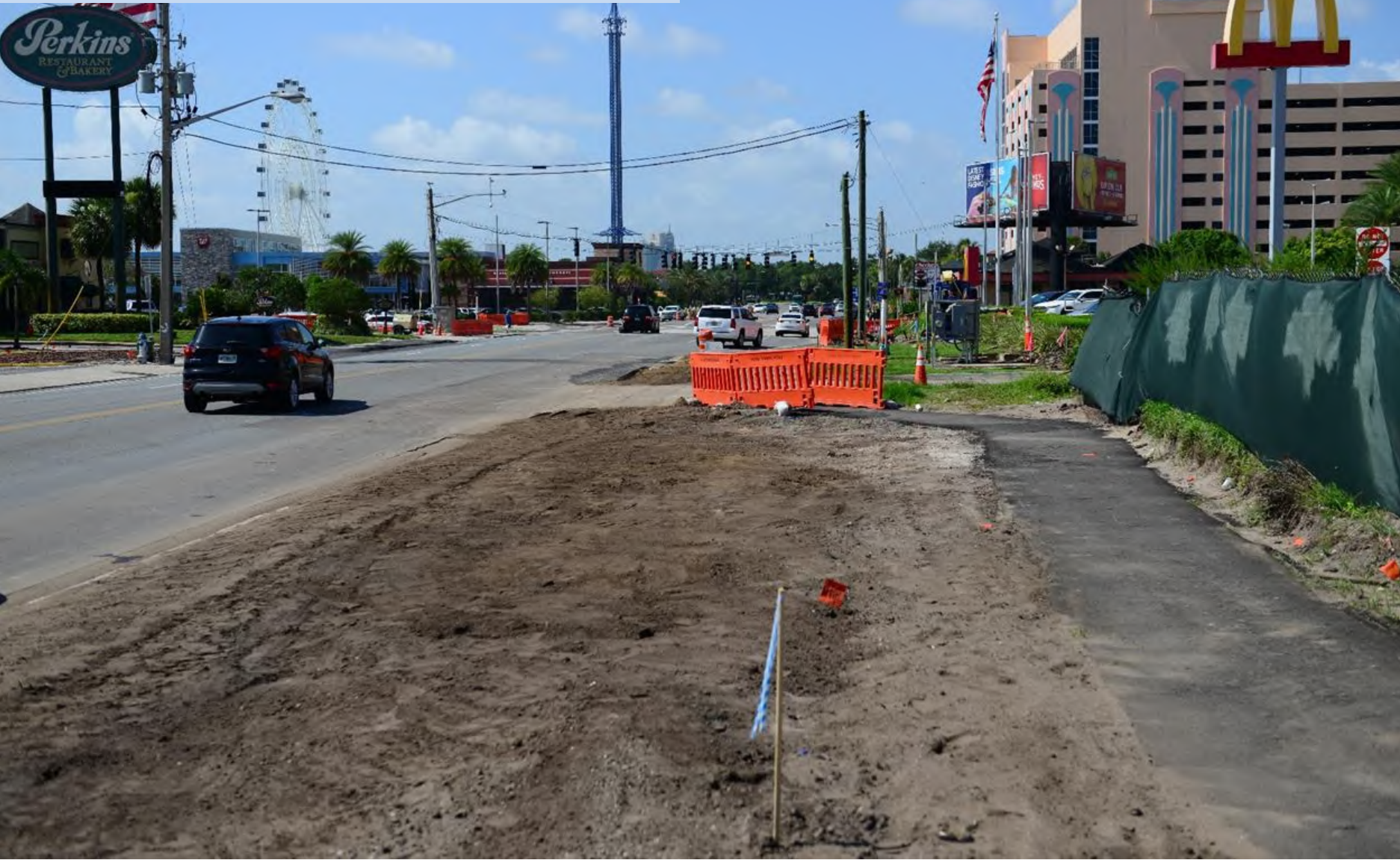
Sidewalk on north I-Drive near McDonald's
