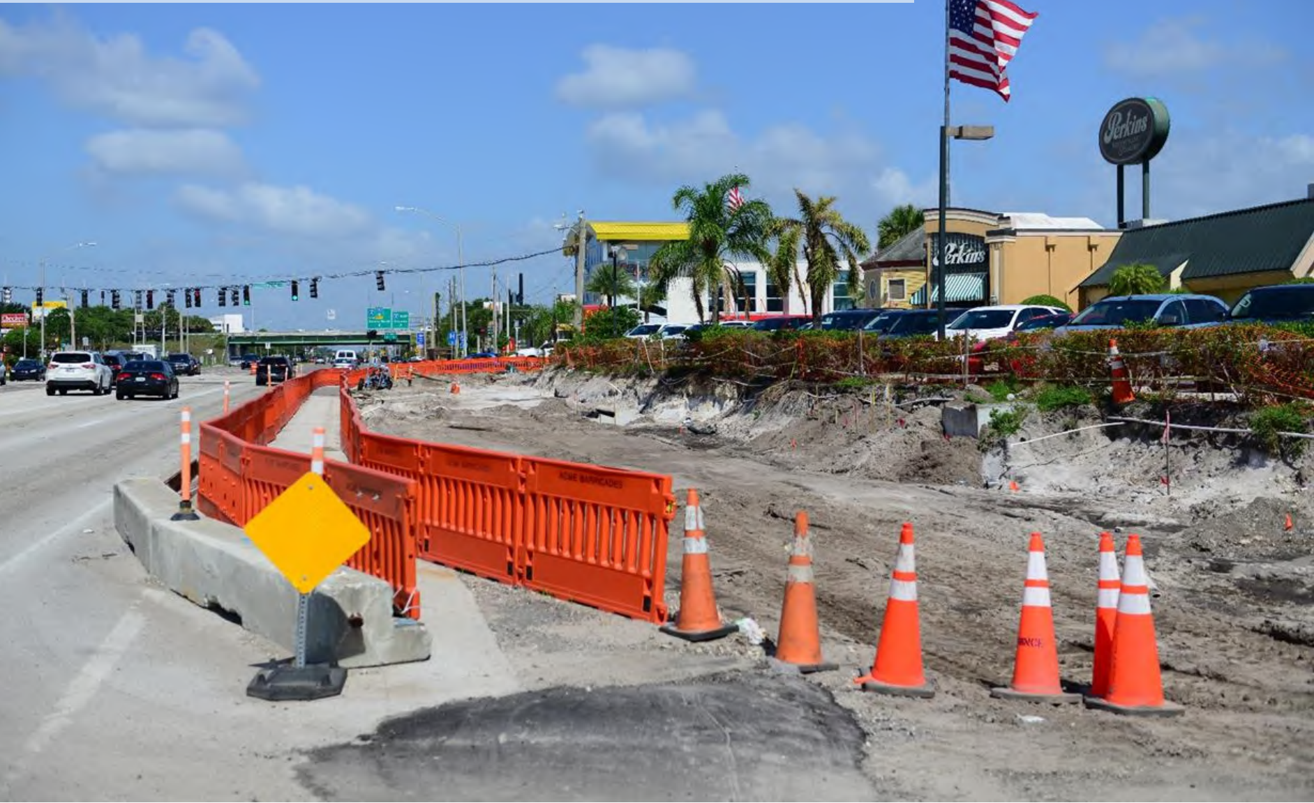
Sidewalk, curb and drainage work on Sand Lake Rd. near I-Drive
