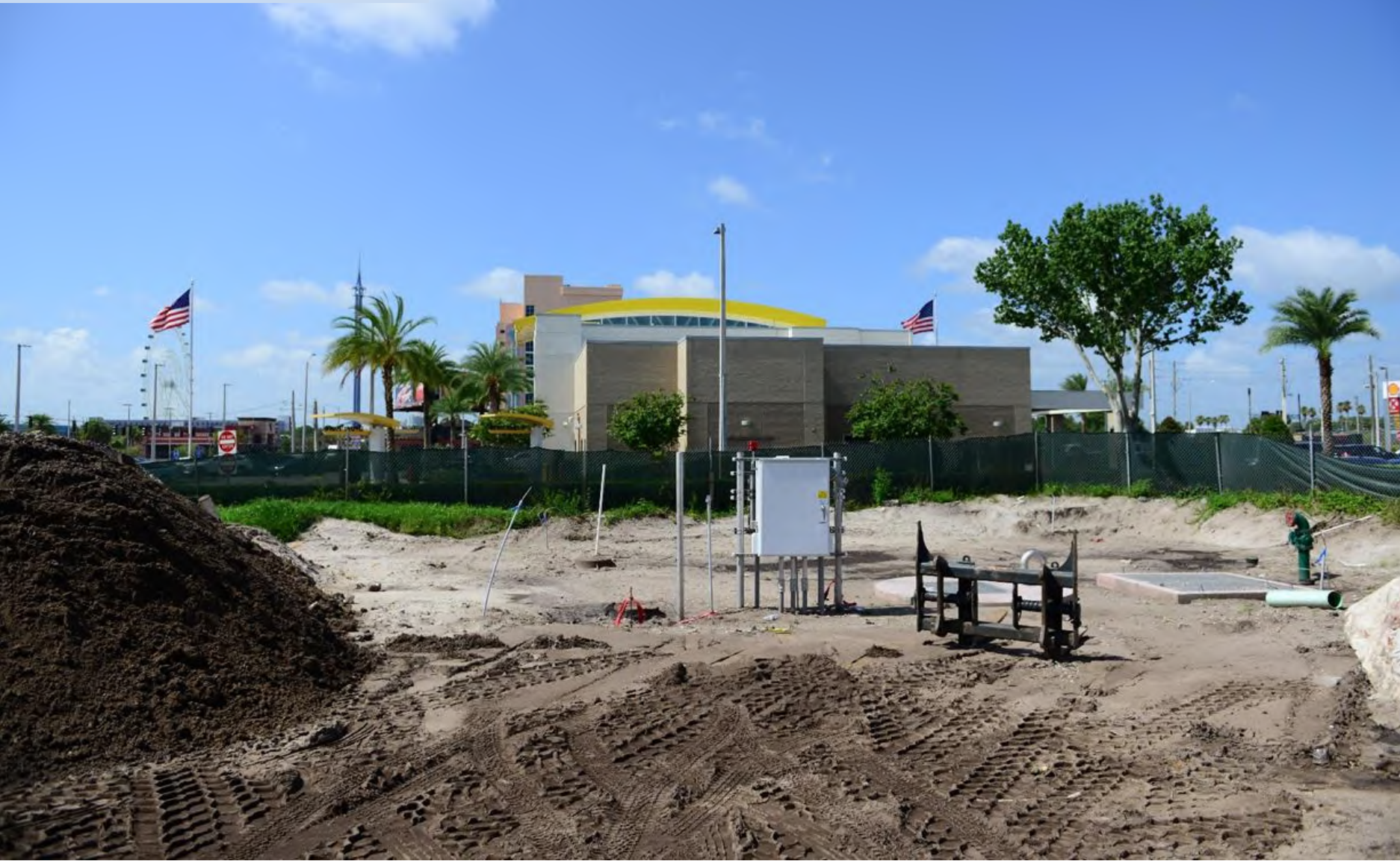
Lift station on north I-Drive
